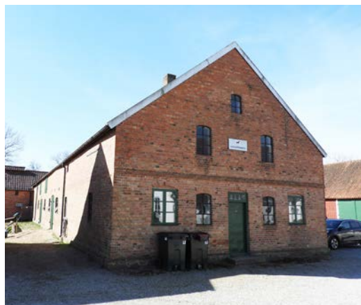
Kostallets gavel mot norr.
